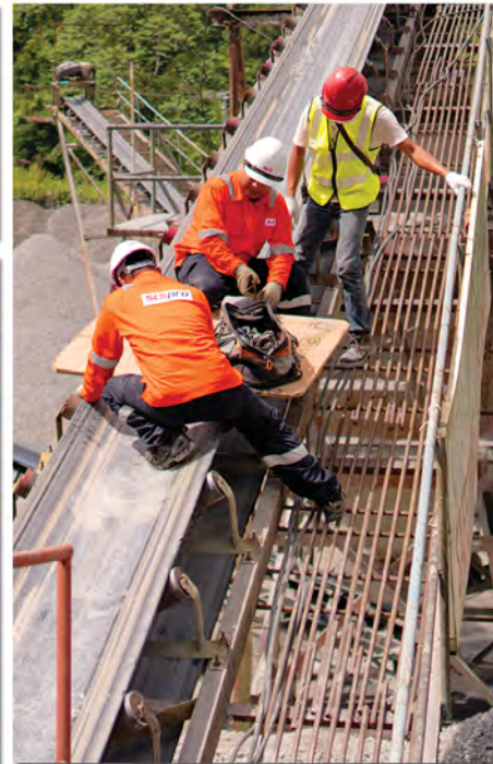
Conveyor Belt Splicing
